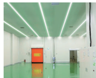
Ceiling panel with built-in LED lights
